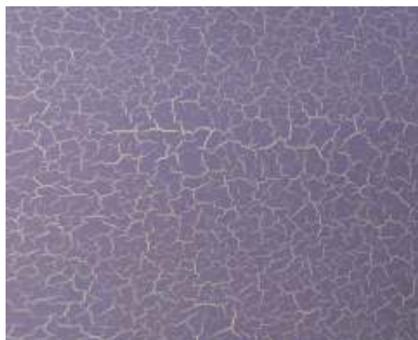
Overpaint by wool roller with coloured 10% diluted water paint (binder content 20%).
